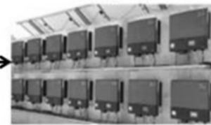
DC/AC converters 28 x 17 kW
